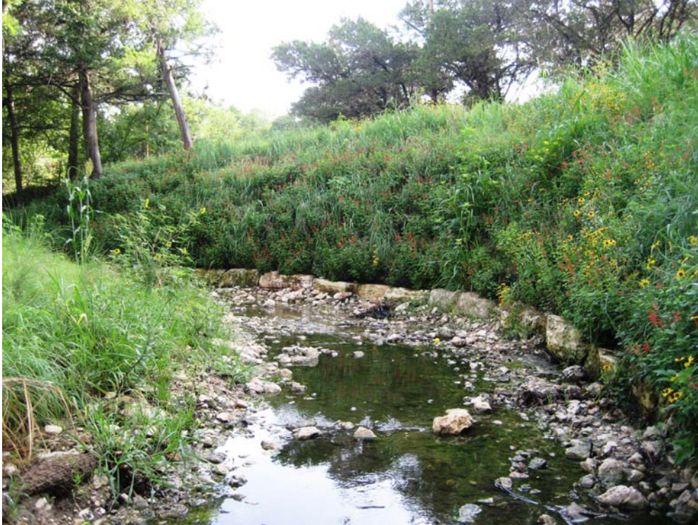
Example Bioengineering Bank Stabilization
