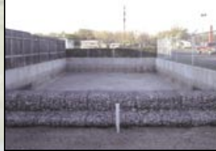
Partial Sedimentation / Filtration Pond
